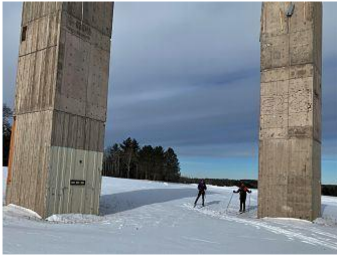
Rita Keber & John Pantazon dwarfed by the giant concrete elevator towers left from Telemark Lodge.
